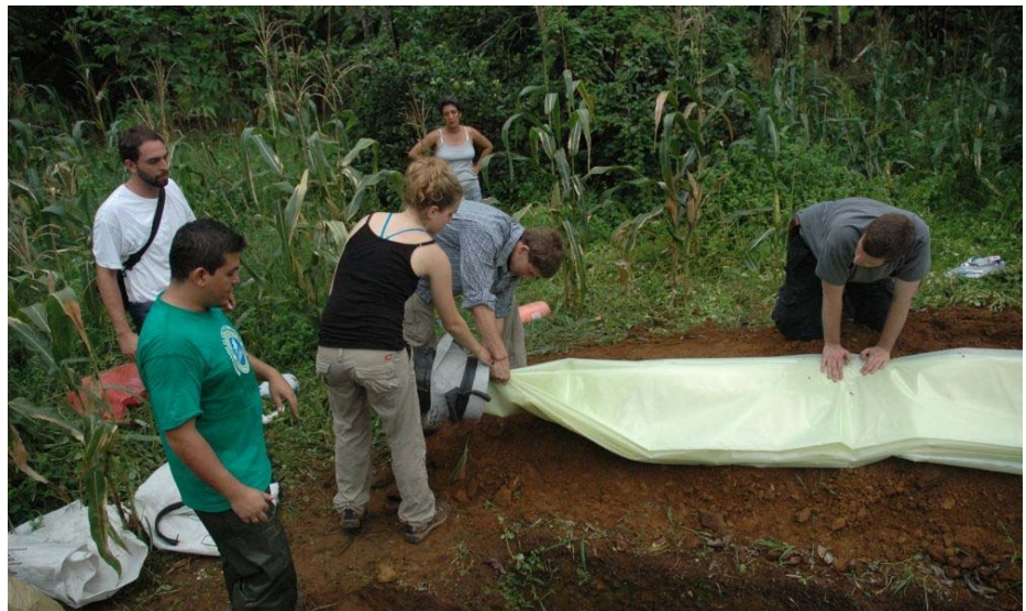
Students in Sustainability of Tropical Ecosystems Field Study assembling a biodigester. Photo by Wayne Parrott
